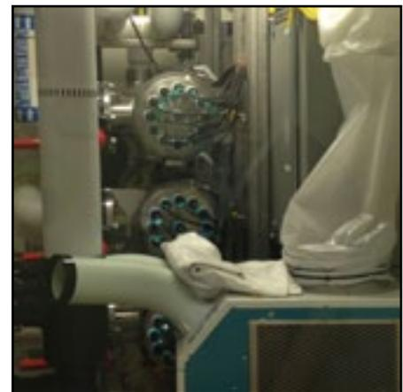
UV filtration is the last stage of treatment. Each of the four stainless steel chambers holds 13 high-intensity UV bulbs.
